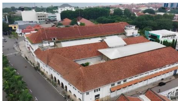
Figure 9. Top View of the BAT Building
