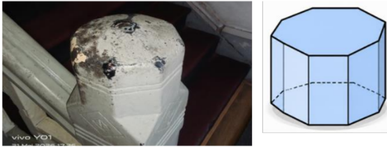
Figure 12. Stair Handrail Ornament
