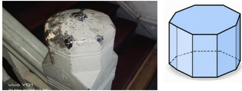
Figure 12. Stair Handrail Ornament
