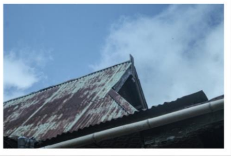
Figure 6. Buwun Sikon Sakok Manu Ladon roof structure
