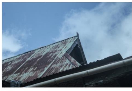
Figure 6. Buwun Sikon Sakok Manu Ladon roof structure
