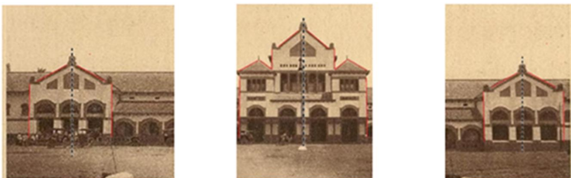
Figure 3. The application of geometric reflection on the façade of the Cirebon Kejaksaan's Station can be seen in the left-center-right division of the structure and the symmetry of the elements of doors, windows, and arches.
