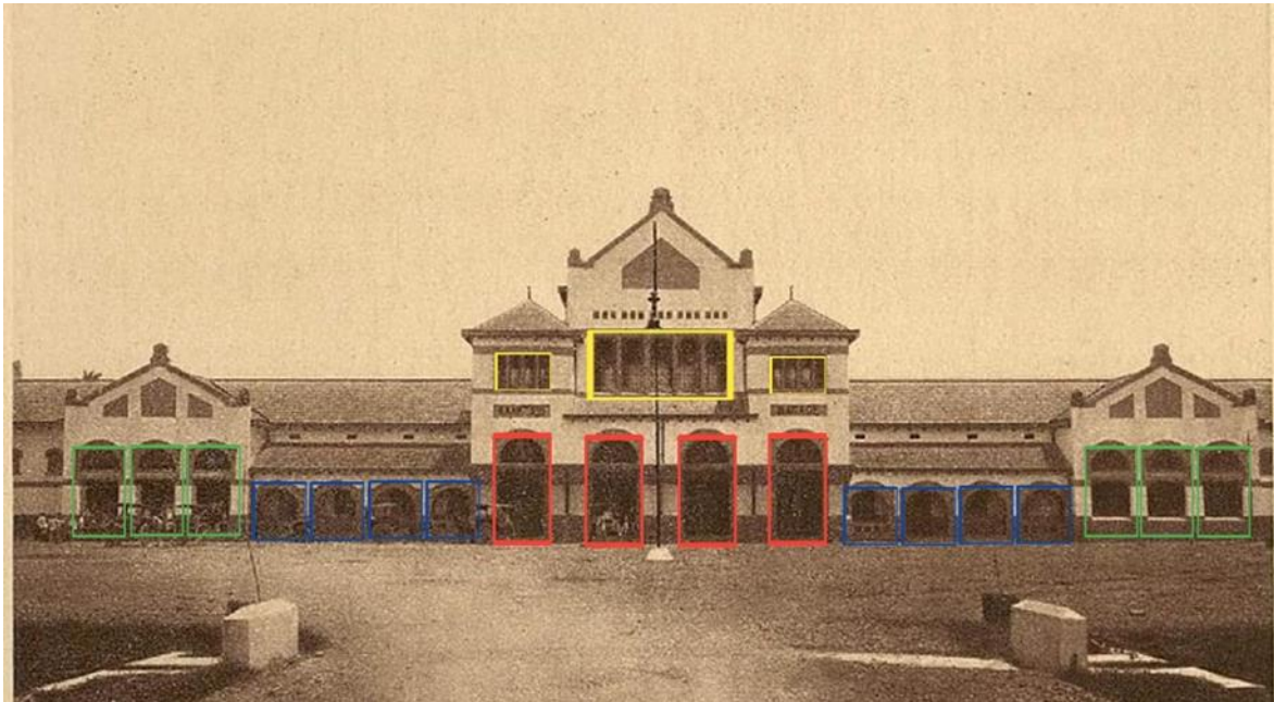
Figure 4. The application of geometric transformation in the form of translation and dilation on the front view of the Cirebon Kejaksaan's Station, which forms the regularity of patterns and proportions of architectural elements
