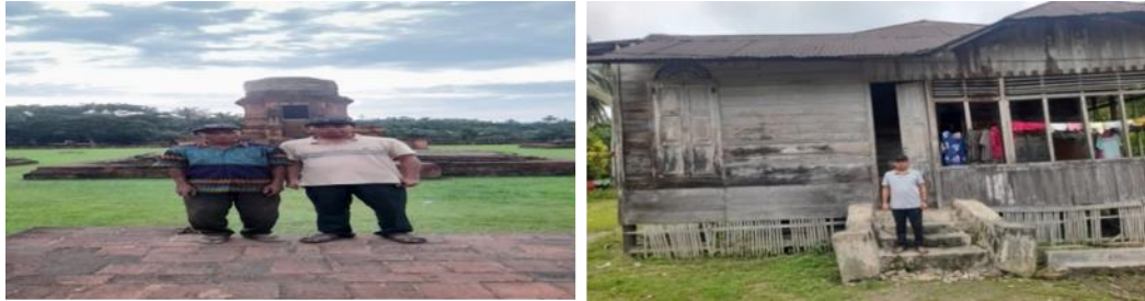
Figure 3. The area of the Bahal Temple or Portibi Temple and the surrounding environment received less government attention
